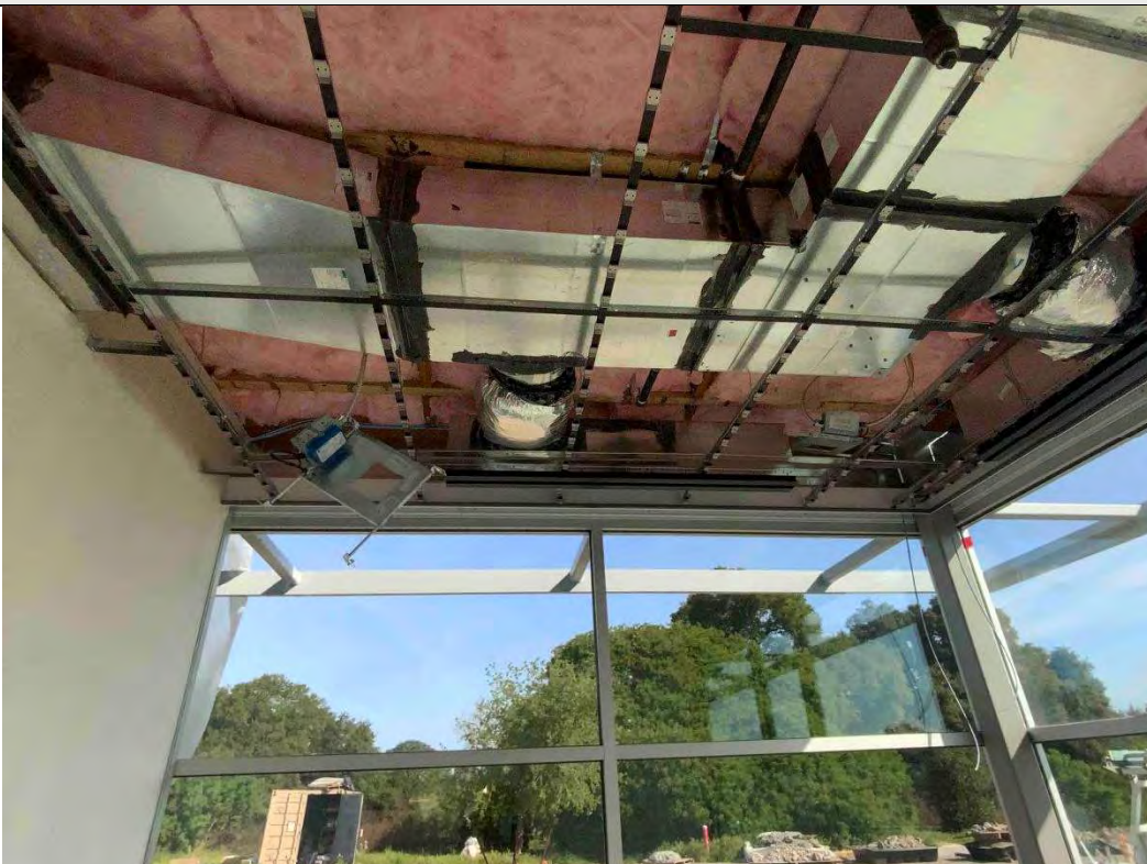
Figure 4: Ducting in Office 107
