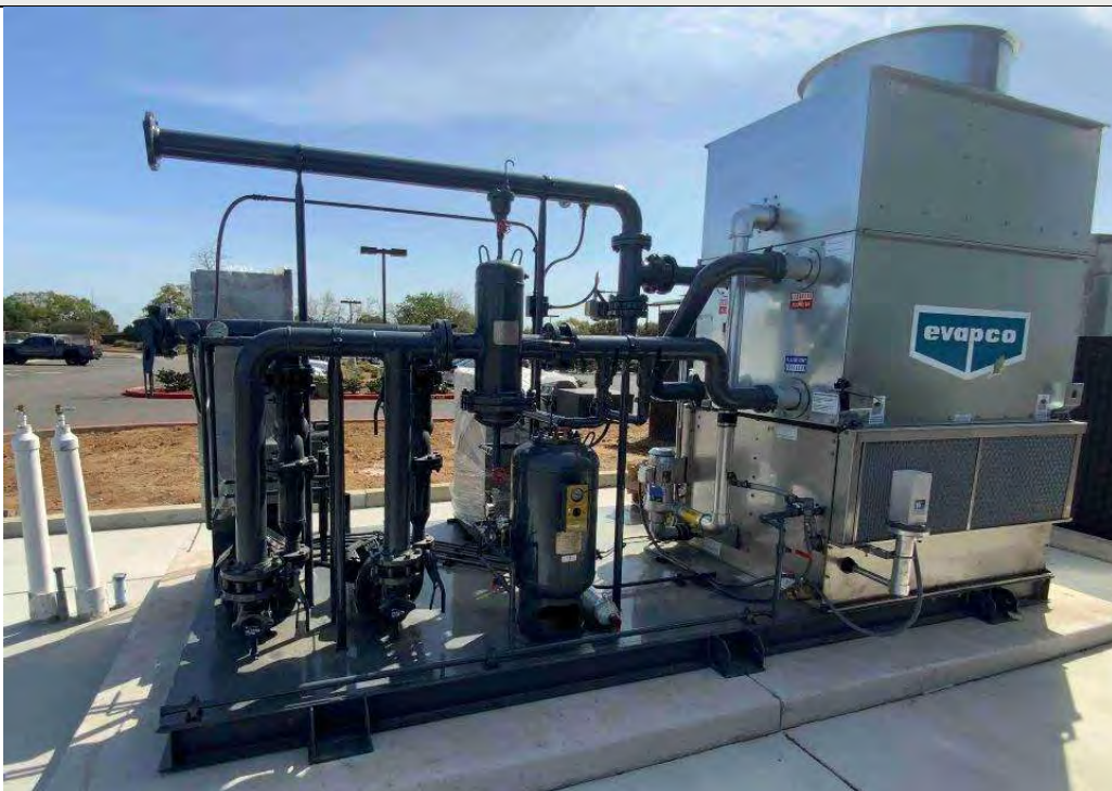
Figure 1: Water Source Heat Pump Skid
