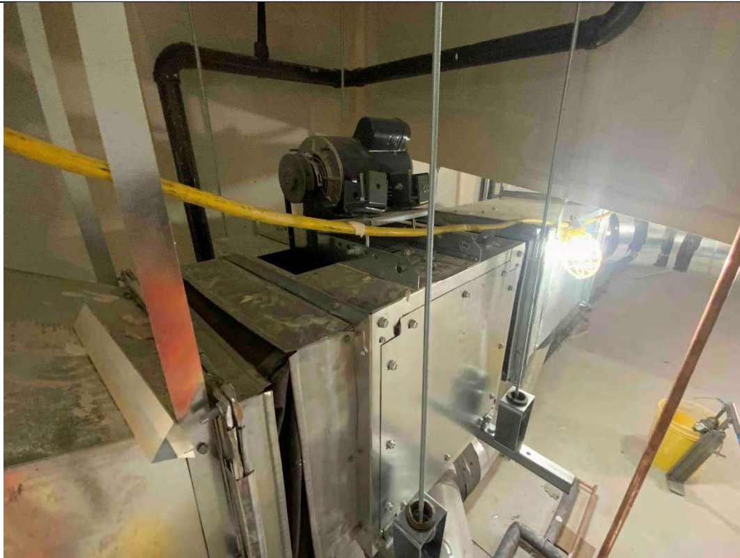
Figure 3: Exhaust Fan
