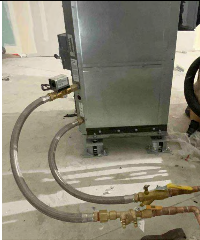
Figure 2: Heat Pump Typical Mounting Installation
