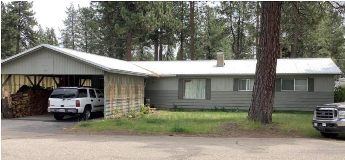
Figure 5-20. North, primary façade of 297 Maywood Drive, view southeast.
