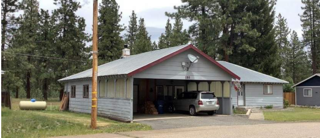
Figure 5-9. South, primary façade of 180 Maywood Drive, view northwest.
