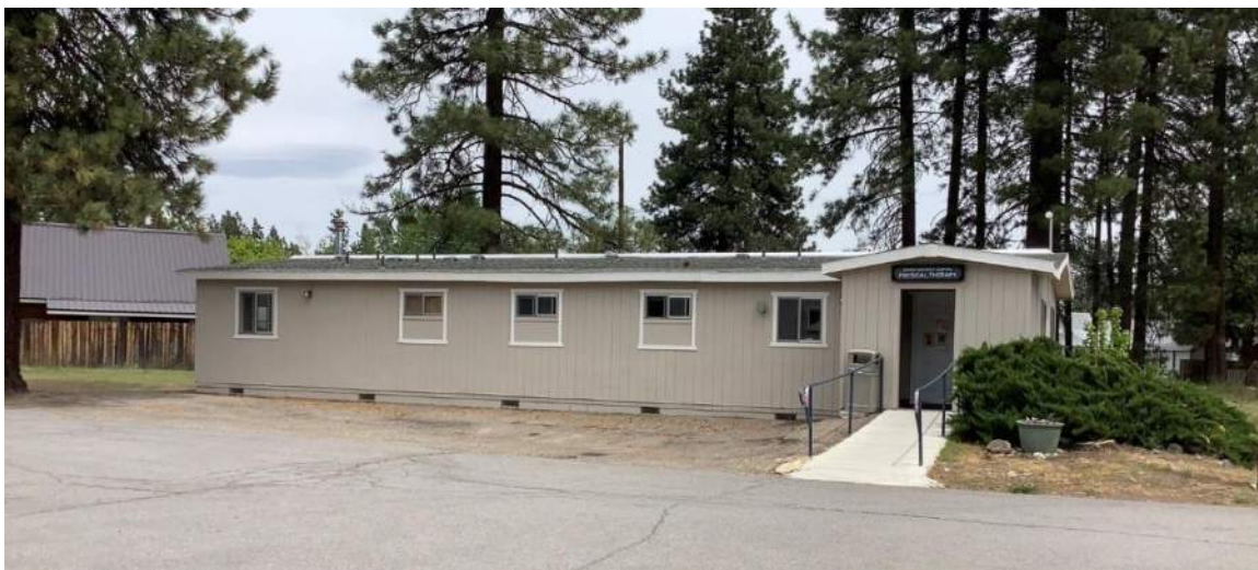
Figure 5-32. West, primary façade of Building 10, 122 Brentwood, camera facing northeast.
