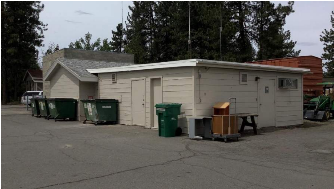
Figure 5-26. View of ancillary buildings from left to right: Building 6, building 2, building 7. Camera facing west.
