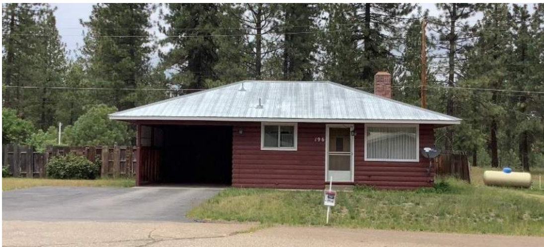
Figure 5-10. South, primary façade of 196 Maywood Drive, view north.
