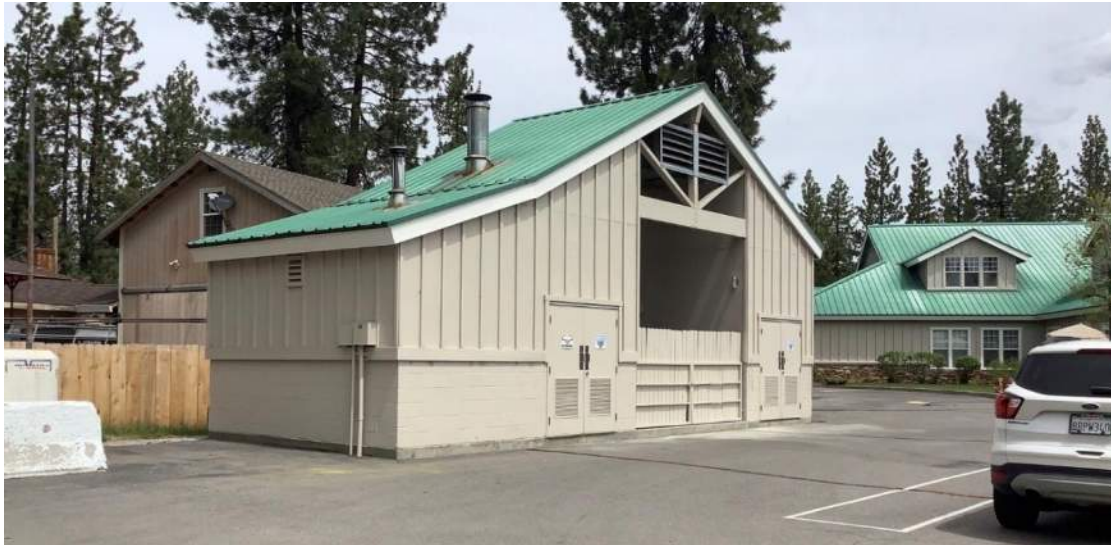
Figure 5-28. East, primary façade of Building 13, camera facing north.
