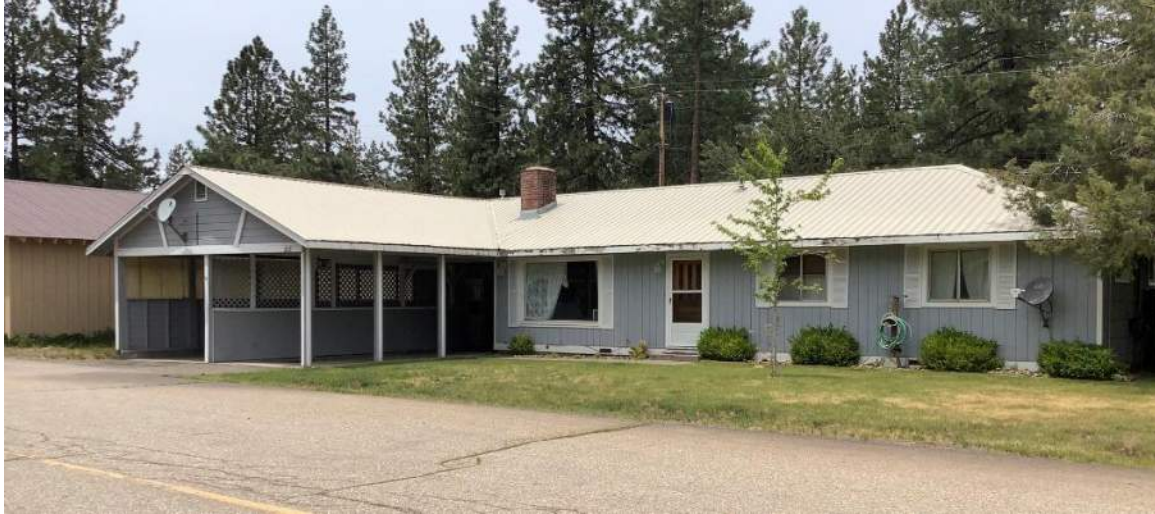
Figure 5-12. South, primary façade of 218 Maywood Drive, view northwest.
