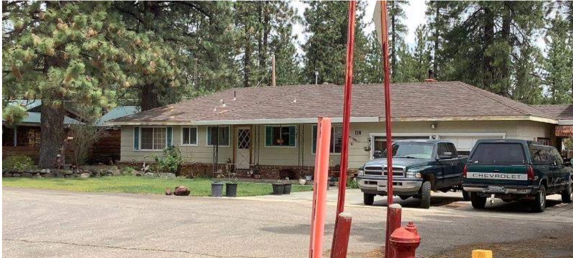
Figure 5-1. West, primary façade of Residence 116, view east-northeast.
