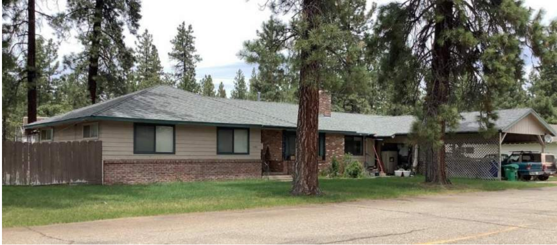
Figure 5-18. South, primary façade of 282 Maywood Drive, view north.
