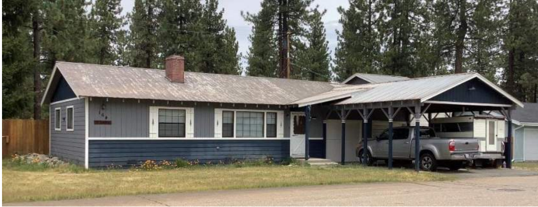
Figure 5-7. South, primary façade of 164 Maywood Drive, view northeast.
