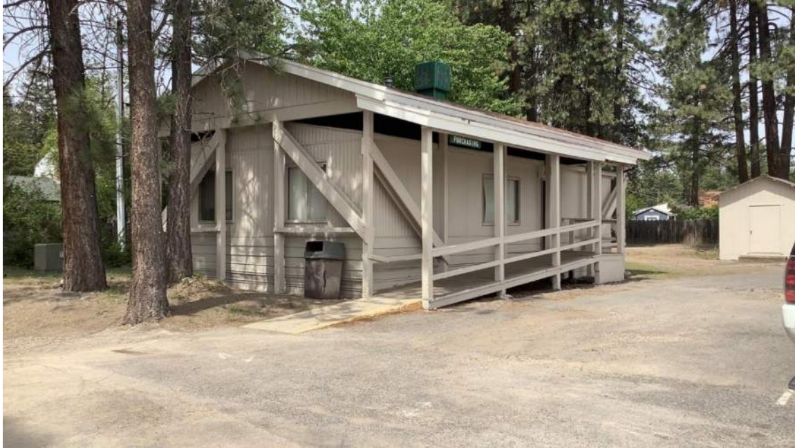
Figure 5-34. East (primary) façade of Purchasing Department Building, camera facing northwest.
