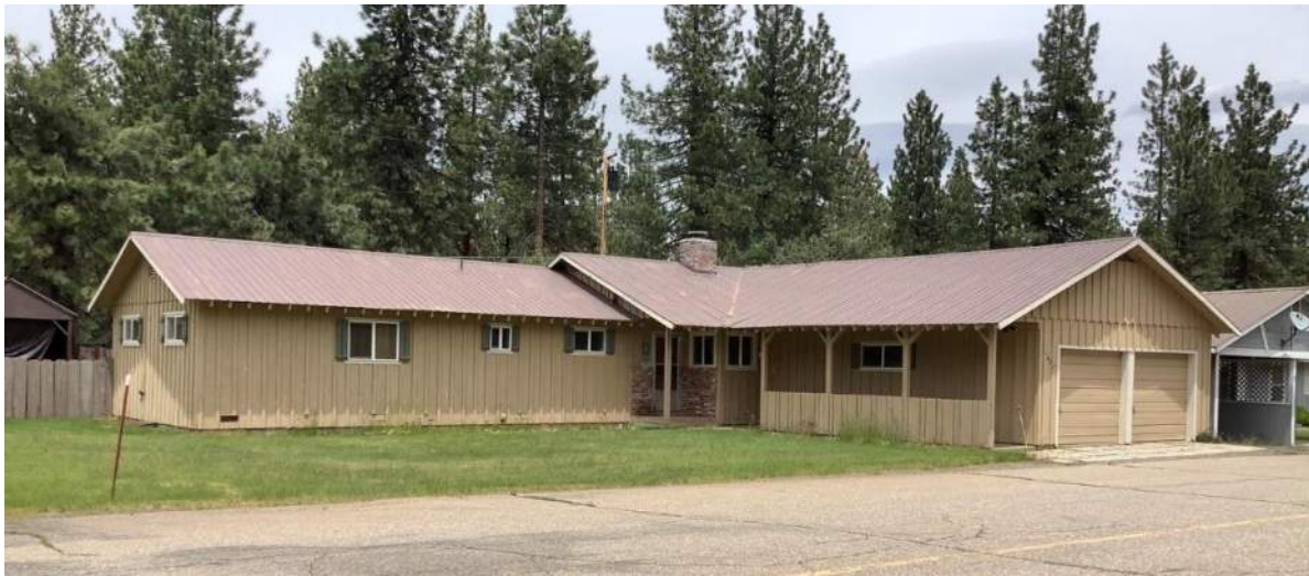
Figure 5-14. South, primary façade of 240 Maywood Drive, view northeast.
