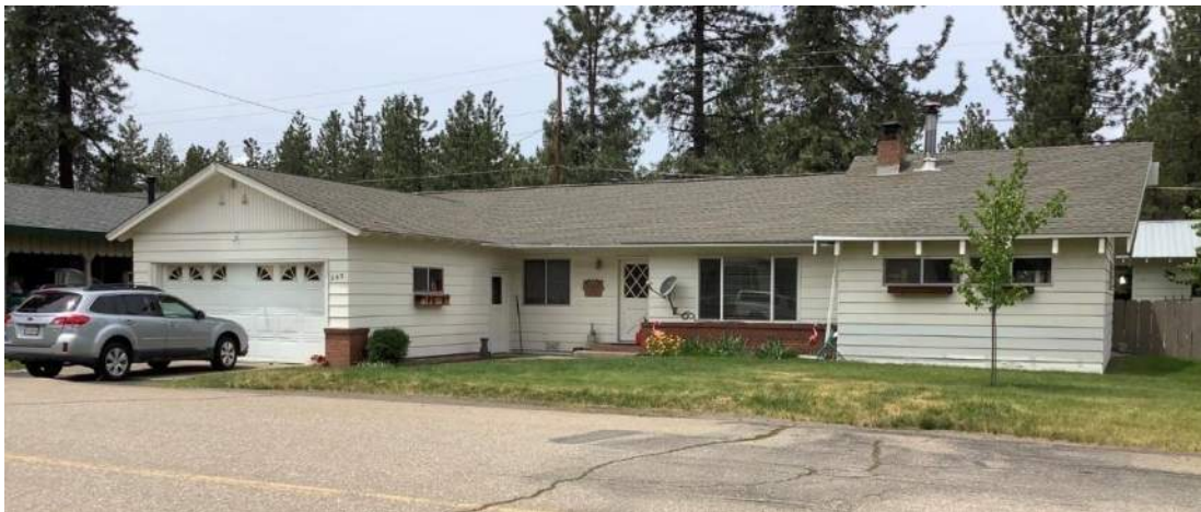
Figure 5-16. South, primary façade of 262 Maywood Drive, view northwest.
