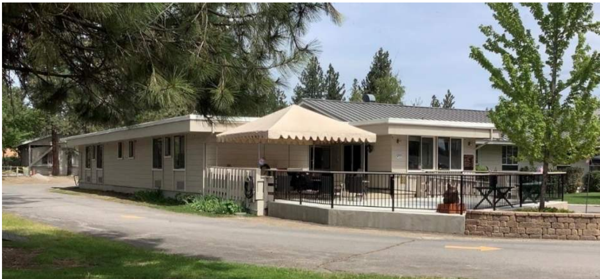
Figure 5-23. Overview of the south and west façades of the Extended Care Addition, view northwest.
