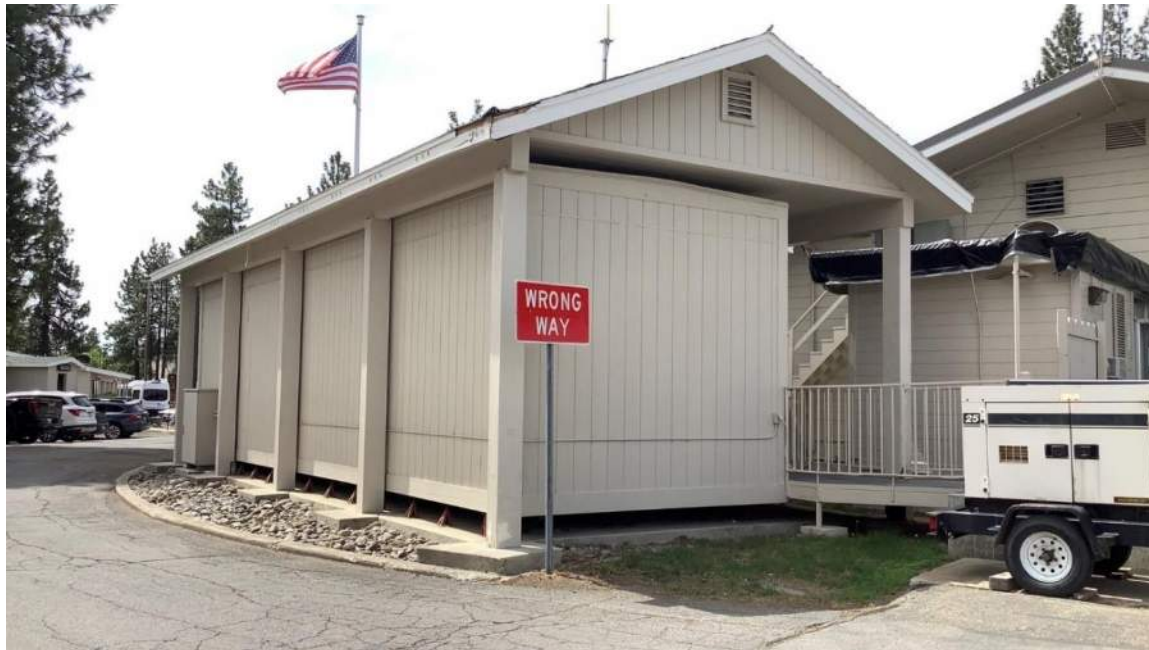
Figure 5-33. West façade of Modular CT building, camera facing east.
