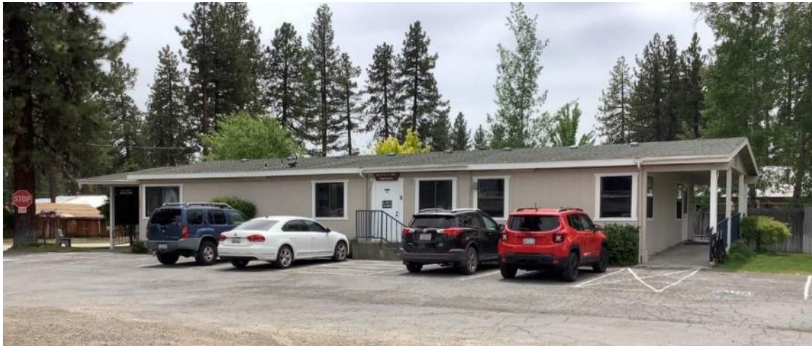
Figure 5-30. Primary, east façade of Building 8 at 150 Brentwood. Camera facing southwest.
