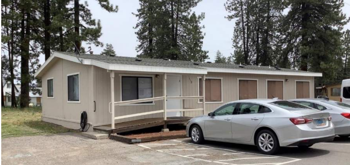
Figure 5-31. Primary façade of Building 9. Staff Housing at 118 Brentwood. Camera Facing east.
