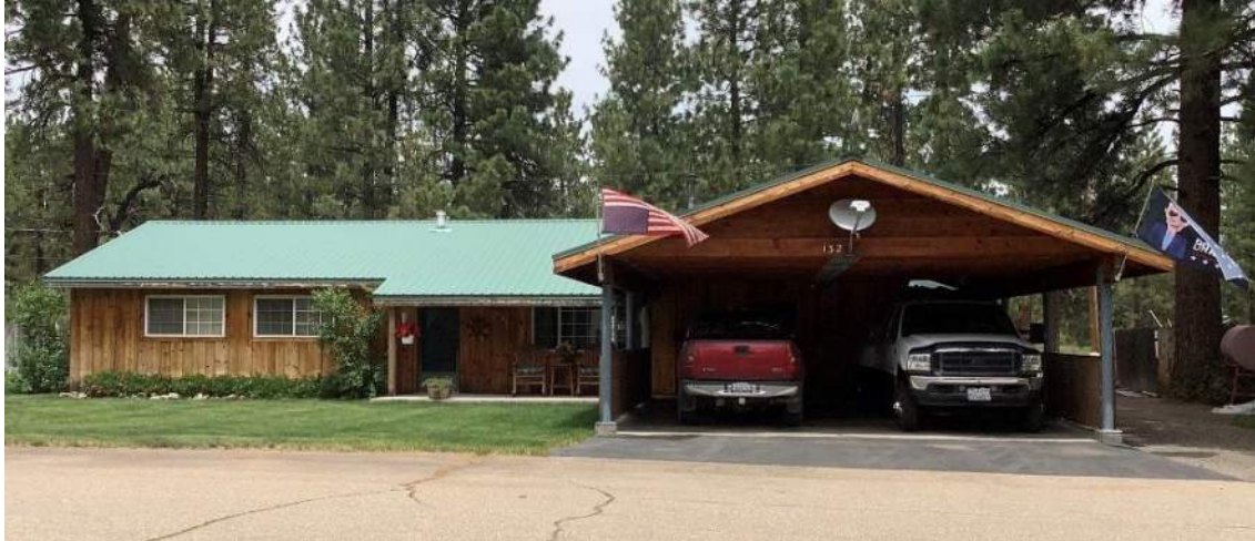
Figure 5-3. South, primary façade of 132 Maywood Drive, view north.
