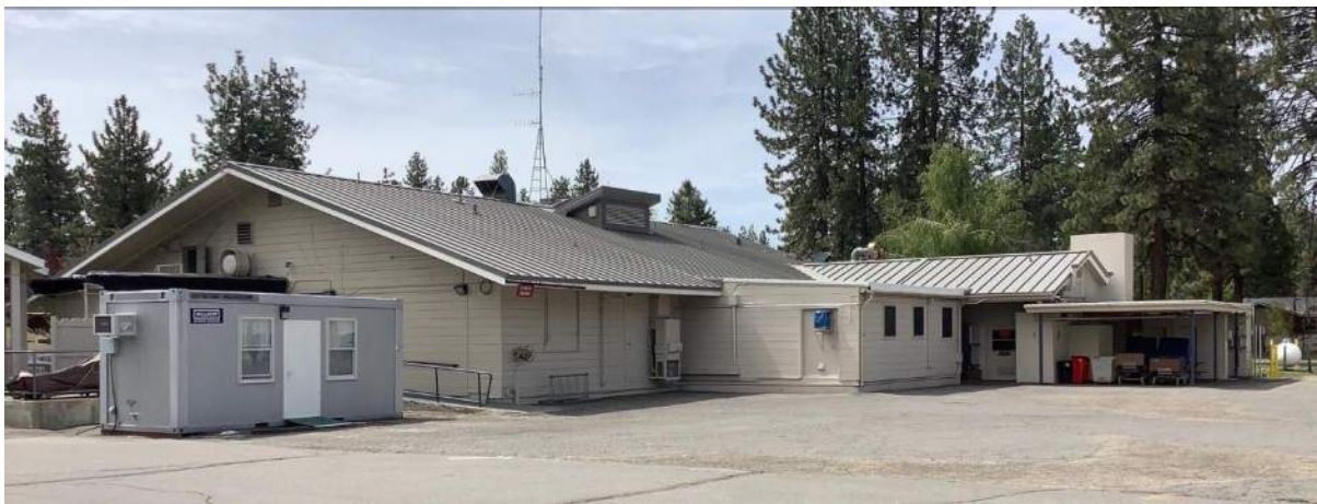
Figure 5-25. North and east façades of the Storage Addition Building, view southeast.
