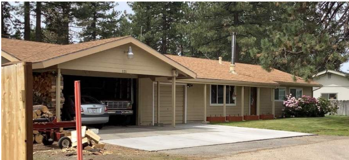
Figure 5-2. North, primary façade of 121 Maywood Drive, camera facing northwest.
