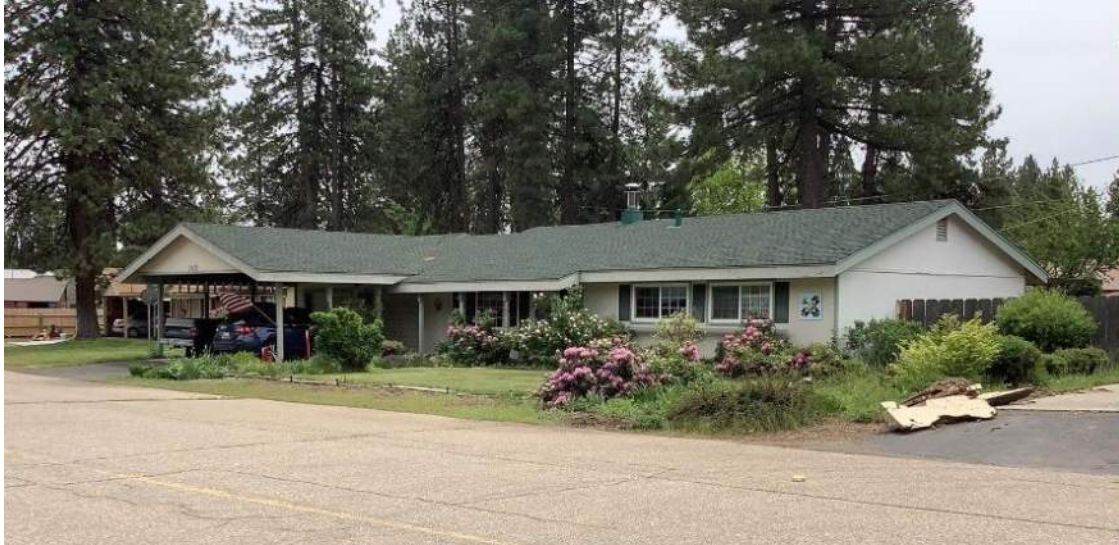
Figure 5-4. North, primary façade of 145 Maywood Drive, view southeast.
