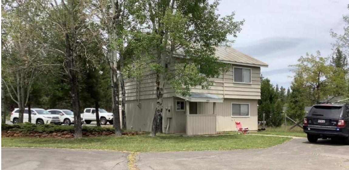
Figure 5-29. East, primary façade of 187 Reynolds Road, camera facing northwest.
